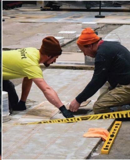
New sections of shiny marble tile are carefully cut to size and installed.
