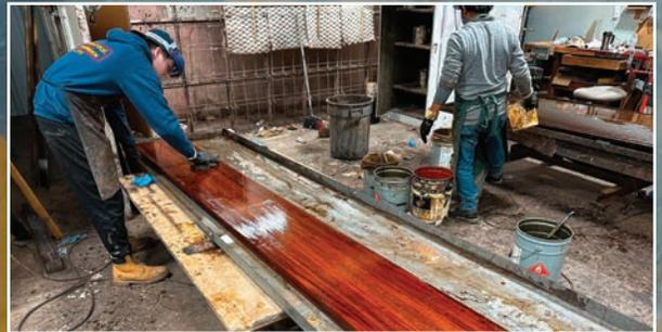
The Basilica pews are stripped of varnish and prepped for extensive sanding and refinishing at Kittinger's facility.
