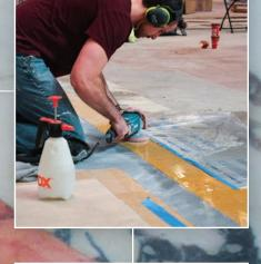
Damaged sections of the floor are carved out and removed, paving the way for replacement marble tile to be installed.
